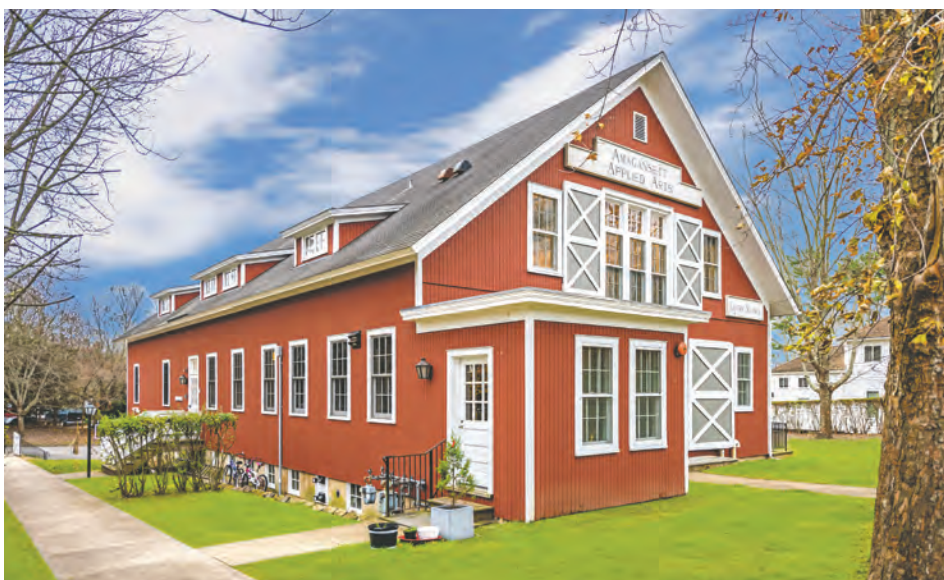
Indian Wells Highway, Amagansett Renovated Commercial Barn Variety of Uses
