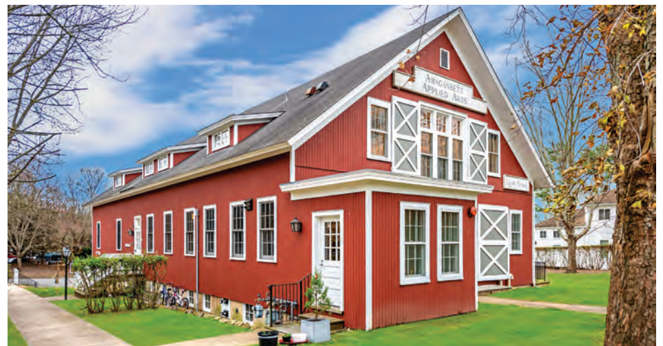
Indian Wells Highway, Amagansett Renovated Commercial Barn Variety of Uses
