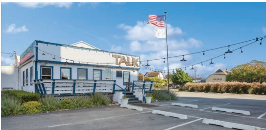
63 South Euclid Road, Montauk Iconic Downtown Restaurant & Bar With Staff Housing. Tremendous Business Potential in a Visible Location.
