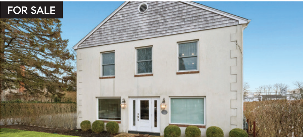
28 Cameron St, Southampton $2,450,000 Freestanding Commercial Building w/ Private Parking, 2,640sf & VB Zoning
